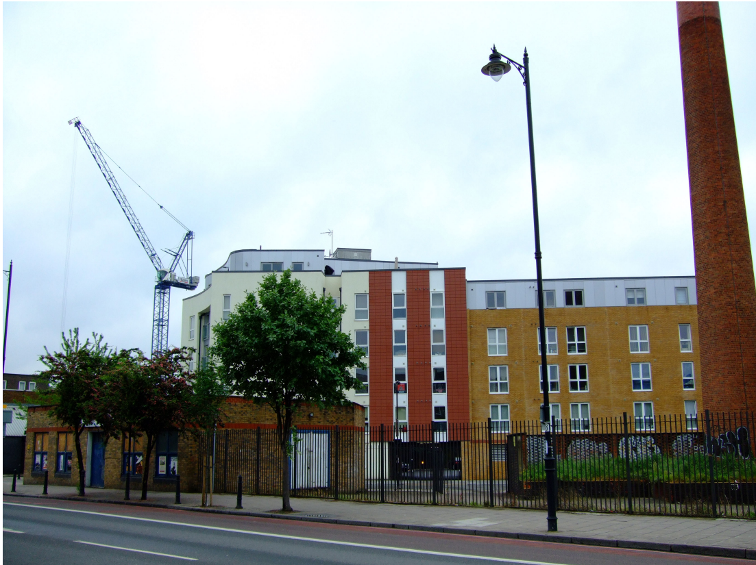
Application site at corner of Kingsland Road and Enfield Road
