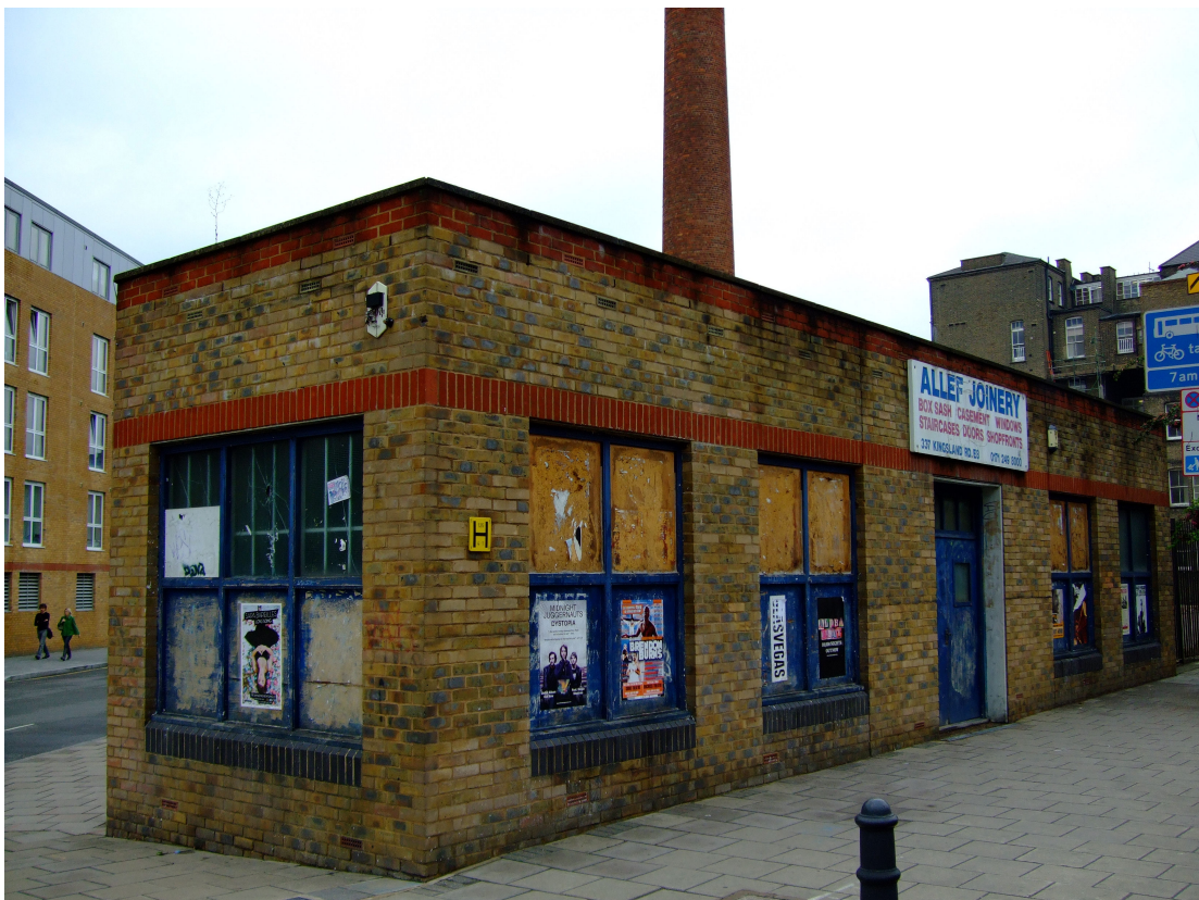
Former joinery building at corner of the application site
